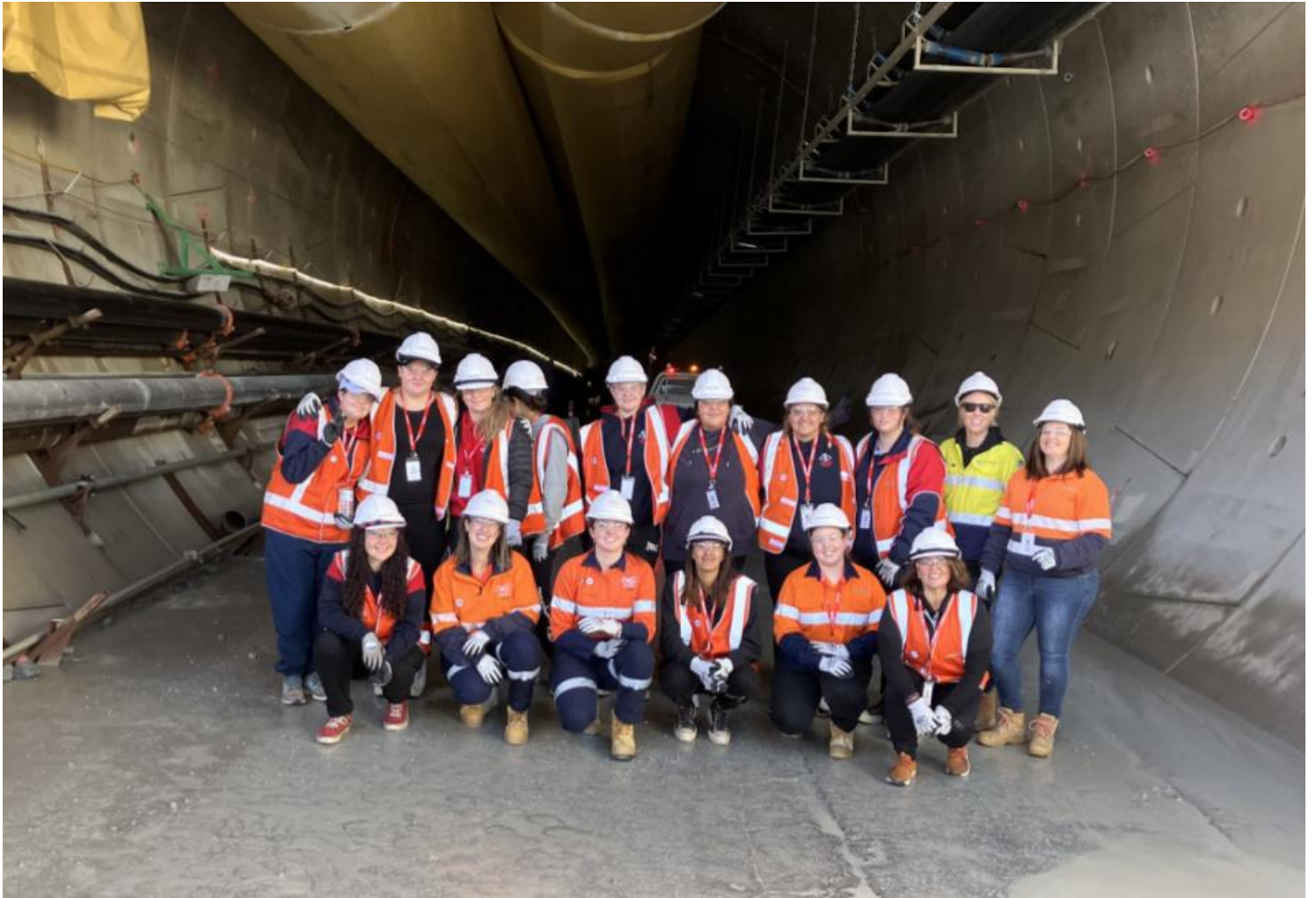
Below: STARS exploring the Tunnel at Lobbs Hole, Snowy Hydro 2.0 Project on 6 th May 2024.
